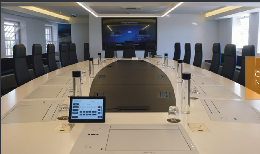
C. M. CASCAIS BOARD ROOM SOLUTIONS | SPECIALIZED TECHNICAL INSTALLATIONS
