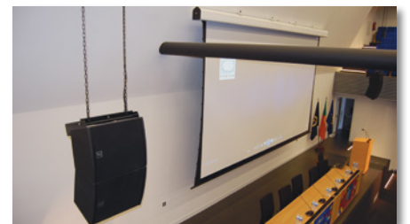
OCC - PORTO SPECIALIZED TECHNICAL INSTALLATIONS
