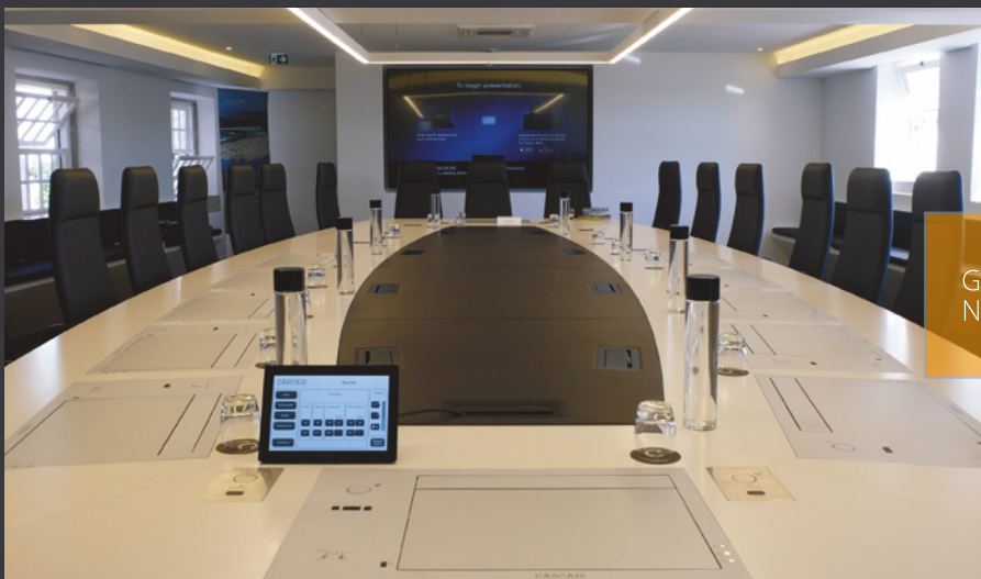
C. M. CASCAIS BOARD ROOM SOLUTIONS | SPECIALIZED TECHNICAL INSTALLATIONS
