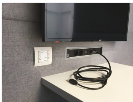
VESTAS CONTROL & AUTOMATION
