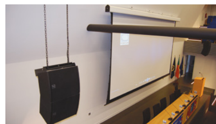
OCC - PORTO SPECIALIZED TECHNICAL INSTALLATIONS
