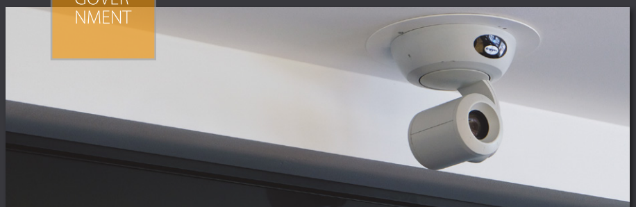
C. M. CASCAIS SIGNAL MANAGEMENT, DISTRIBUTION AND ROUTING | SPECIALIZED TECHNICAL INSTALLATIONS
